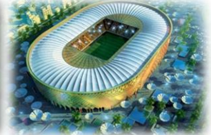
8. Qatar University Stadium Capacity: 43,520 Value: US$ 300 mn
