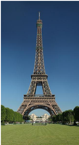
Eiffel Tower: 319m high, 7,300tonnes of steel (wrought iron)
