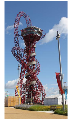
ArcelorMittal Orbit: 115m high, 1,400tonnes of steel
